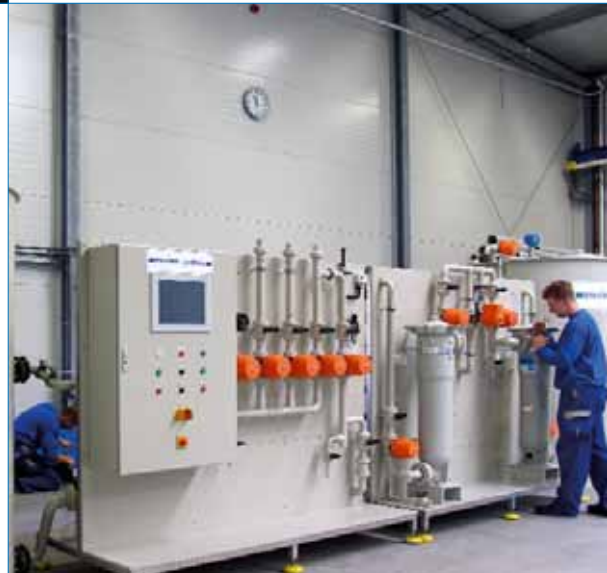
Montage in Rossdorf Assembly in Rossdorf
