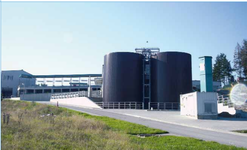
aerobe Membranbiologie BIOMAR® OMB zur Behandlung von Deponie-Sickerwasser aerobic membrane bioreactor BIOMAR® OMB for the treatment of landfill leachate
